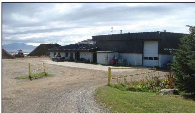
City of Homer existing Public Works facility.
