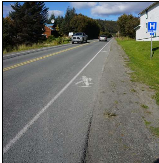
Pedestrian safety along Main Street, one of Homer’s primary north-south roads, would benefit from a sidewalk facility.
