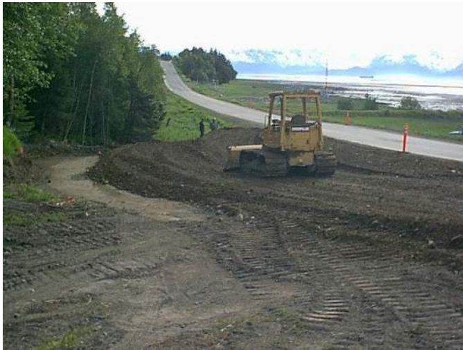
Photo 14: Fill placement for parking lot "A" (6/18/99)
