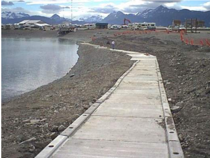
Photo 36: South end of Fishing Hole HC Pathway at low tide. Note that at high tide most of the precast section is flooded. (7/29/99)
