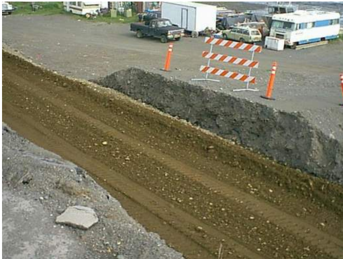
Photo 8: Fill across driveway at Sta 7+995. Compare with 6/11/99 photo #10. (6/18/99)
