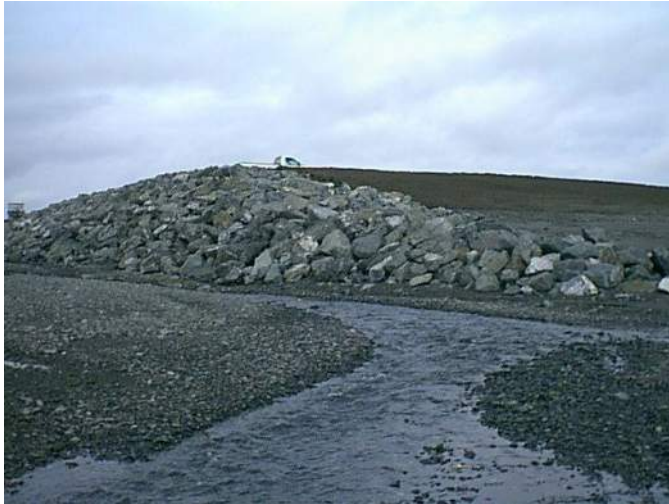
Photo 3: Completed berm extension at Fishing Hole as viewed from bay side. Note fresh earthwork behind rip rap. (5/28/99)
