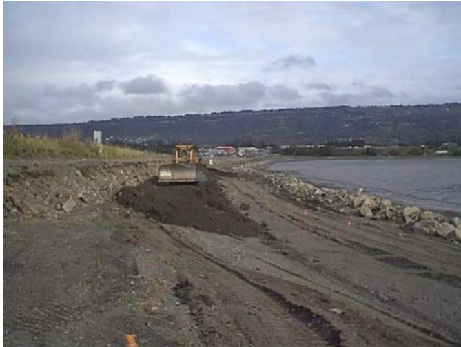
Photo 9: Grading & benching for truck haul route. (5/28/99)
