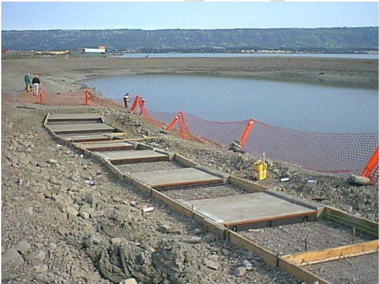
Figure 3. Poured concrete during the initial build of the access ramp in 1999
