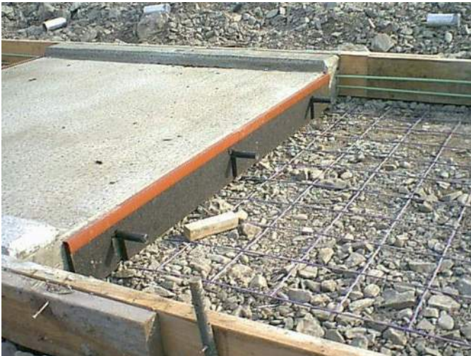
Photo 31: Detailed view of doweled joints (7/9/99)
