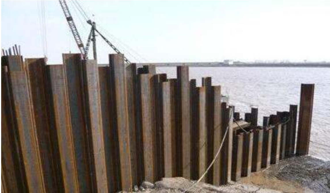
Figure 11. Example of steel sheet pile; piling used along the path would be sized, trimmed, and capped to create a cleaner look than shown in this image (Source: https://www.sheet-piles.com )
