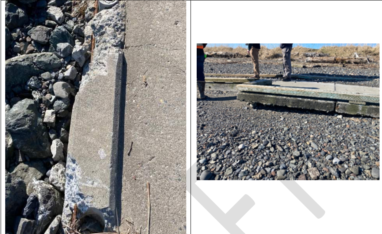
Figure 5. Existing ramp damage at the Homer Fishing Lagoon
