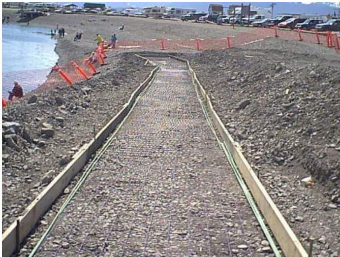
Photo 21: Formwork for south end of Fishing Hole pathway (6/25/99)
