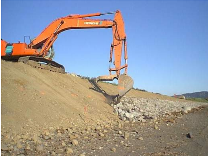
Photo 11: Placement of rip rap along pathway side slope, typ. Contractor spent first half of week pulling fat slopes in this area, working from top of pathway grade with this excavator, as shown. (7/2/99)
