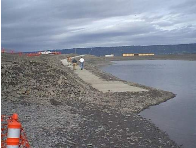
Photo 34: All precast sidewalk panels have now been placed for the Fishing Hole HC Pathway. Cast-in-place concrete work has also been completed. (7/29/99)
