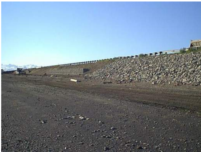
Photo 12: Rip rap slope and gabion wall between Sta. 7+250 & Sta. 7+480 (7/2/99)
