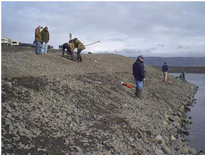
Photo 4: Fishing Hole bank along proposed pathway grade. Note that rip rap seen in earlier photos of this area has now been covered with 2" minus material. This material was obtained from the "undersize" pile at the rip-rap screening yard. (5/28/99)
