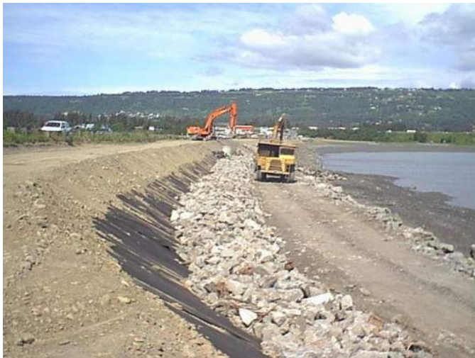
Photo 25: Another view of fresh riprap on slope, looking north from Sta. 6+825 (6/25/99)
