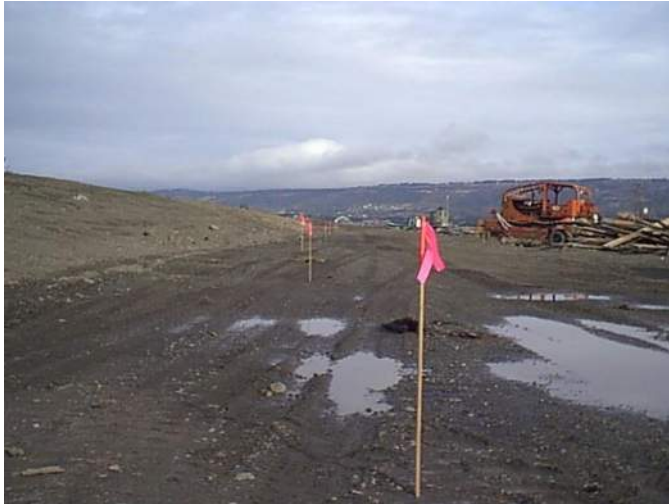
Photo 7: Typical pathway slope staking. This was a major activity of the week, with toe-of-slope stakes placed from H.T.I.'s yard back to Kachemak Bay Drive. (5/28/99)
