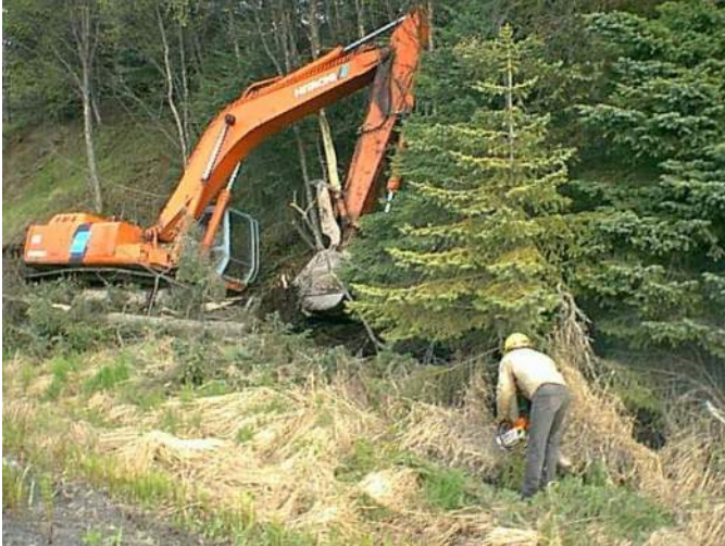
Photo 11: Clearing & grubbing for parking lot "A", at corner of K. Bay Dr. & Homer Spit Rd. Note that backhoe is stuck in the mud. Existing material in ditch is quite soft. (5/28/99)
