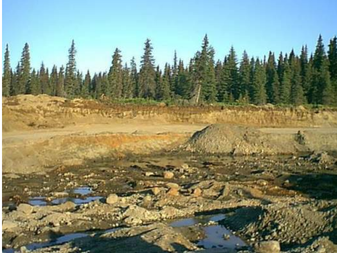
Photo 28: The area of the pit which has been mined for Borrow "A". Most of the pathway is up to grade. Hauling of borrow is about done. (7/2/99)
