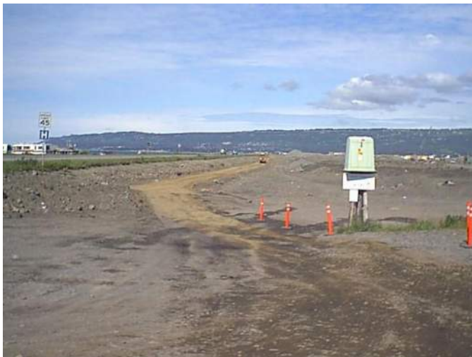
Photo 23: Fill placement for pathway embankment has now progressed as far south as the Fishing Hole parking lot. At the end of the day (Friday, 6/25), 82,000 metric tons of fill had been placed (121% of plan quantity for Borrow "A"). Contractor will not be hauling again until Wednesday of next week. Monday & Tuesday will be spent reshaping previously-placed material.
