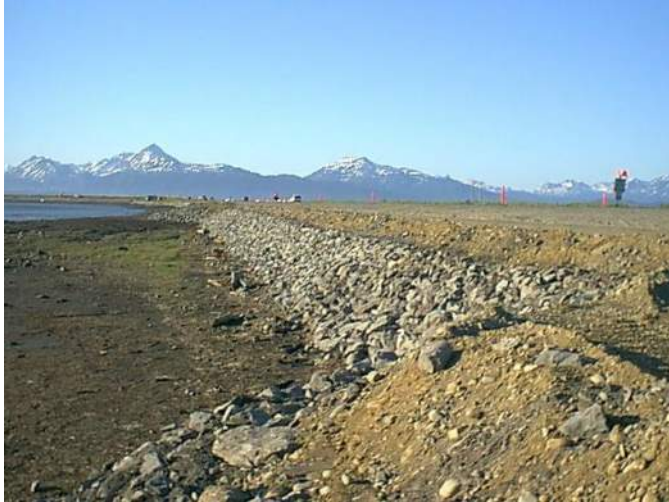
Photo 5: View of rip rap on pathway side slope, looking south from scenic viewpoint at Sta. 6+180. (7/2/99)
