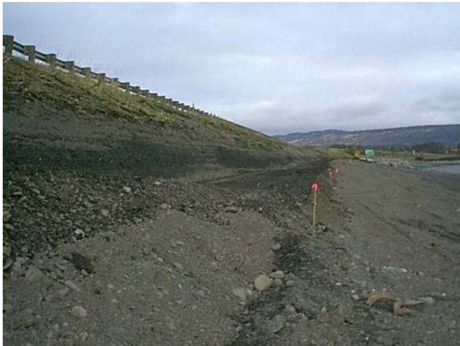
Photo 8: Typical grading & benching construction for truck access during pathway fill operation. Contractor intends to use belly-dumps w/ pup trailers ("Doubles") for haul run from Brown's Pit in Anchor Point. (5/28/99)
