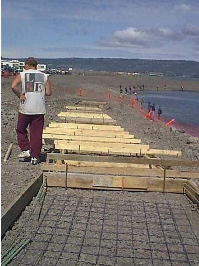
Photo 20: Formwork for north end of Fishing Hole pathway (6/25/99)
