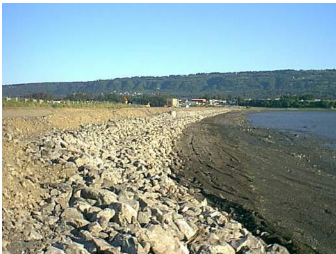
Photo 6: View of rip rap on pathway side slope, looking north from Sta. 6+825. Compare with Photo 6 from last week's set of pictures. (7/2/99)
