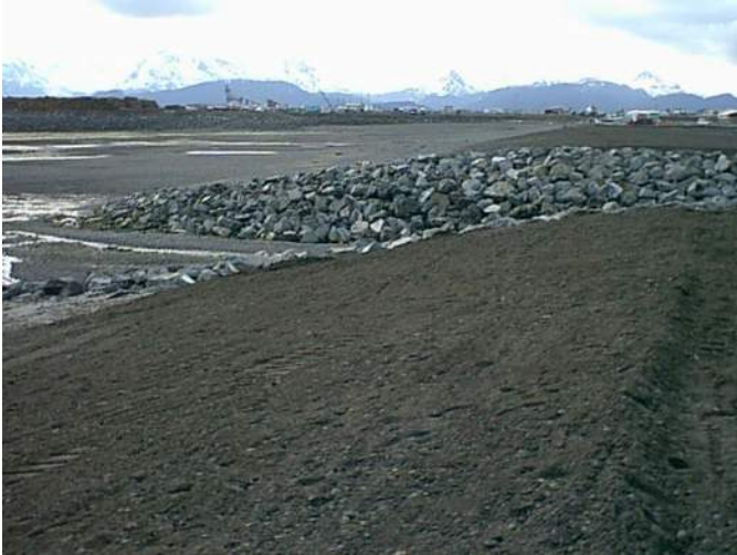
Photo 1: Completed berm extension at Fishing Hole inlet. (5/28/99)
