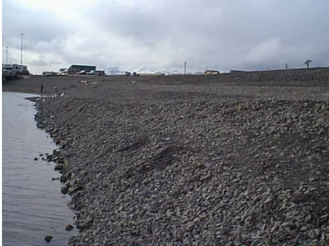
Photo 5: Another view of 2" minus material placed over rip-rap on Fishing Hole pathway embankment. (5/28/99)
