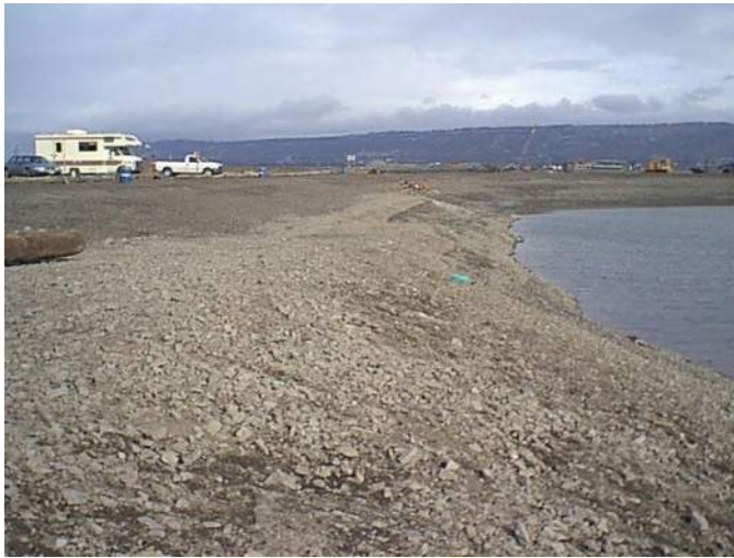
Photo 6: Grading work for concrete pathway at Fishing Hole. (5/28/99)
