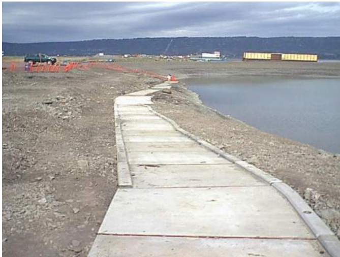
Photo 35: North end of Fishing Hole HC Pathway at low tide. Note that at high tide most of the precast section is flooded. (7/29/99)
