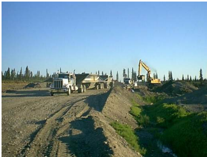
Photo 27: Loading of Borrow "A" at Brown's Pit. By the end of Thursday, approximately 88,000 metric tons of Borrow "A" had been placed, 129% of the plan quantity. (7/2/99)
