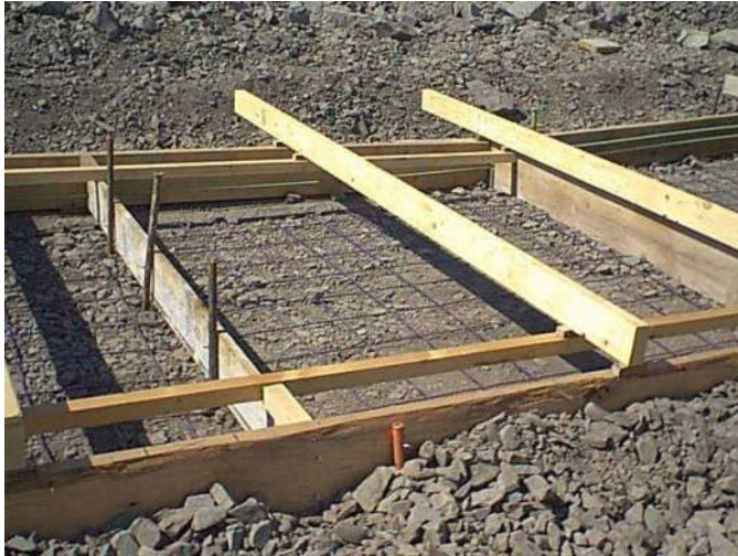
Photo 22: Detail view of Fishing Hole pathway formwork (6/25/99)
