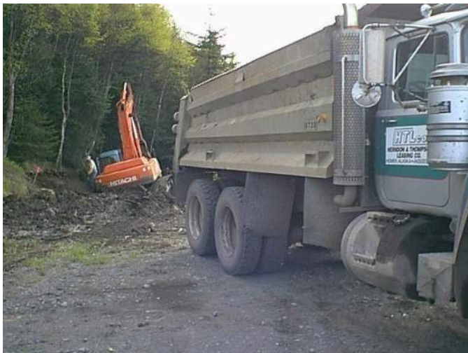
Photo 10: Clearing & grubbing for parking lot "A", at corner of K. Bay Dr. & Homer Spit Rd. (5/28/99)
