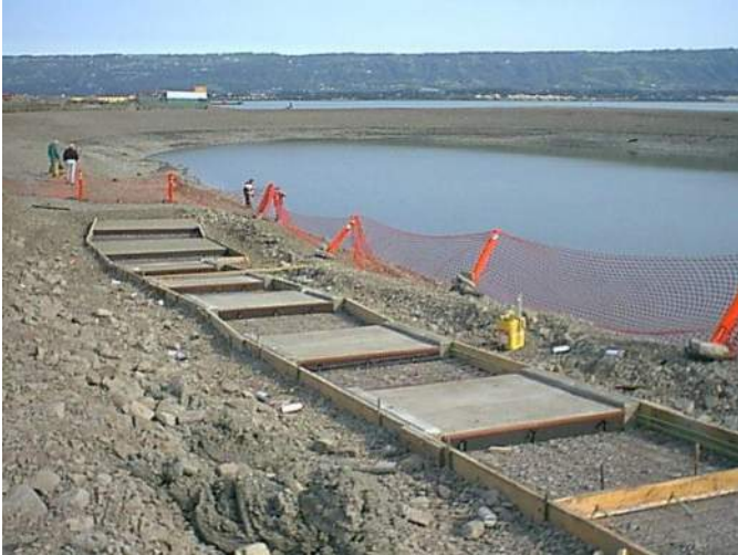
Photo 30: Overall view of Fishing Hole concrete pathway panels which were poured on Thursday. (7/9/99)
