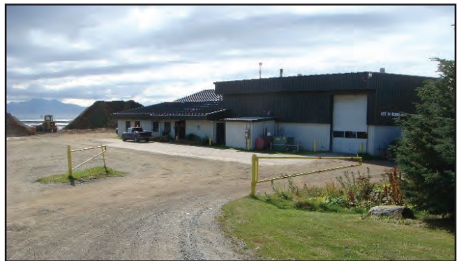
City of Homer existing Public Works facility.
