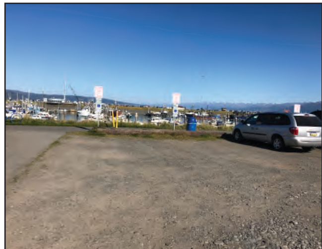
Accessible parking spaces at Ramp 4 in the Port & Harbor provide an example of where spaces need to be paved and a path of travel provided.
