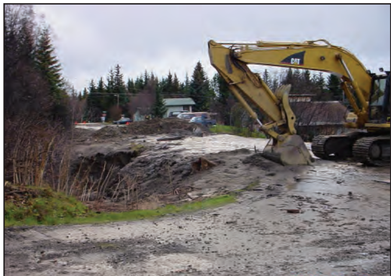
The Slope Stability Program utilizes nature based and low impact development techniques to mitigate erosional damage and protect water quality.
