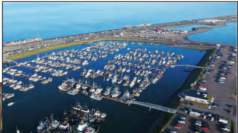
System 4 floats to be replaced.
