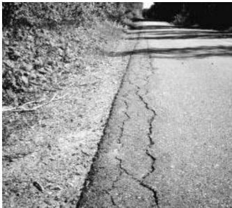
No drainage leads to failed pavement.
