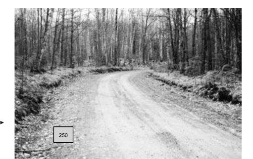
No ditch. Road is actually trenched into roadside forcing water onto surface.
