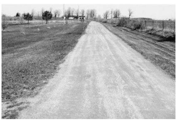
Adequate drainage and fair crown. A few small potholes indicate need for regrading and additional gravel.
