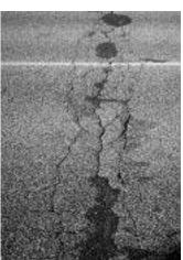
▲ Water enters unsealed cracks softening pavement and Ing secondary cracks.
