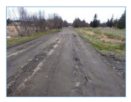
Figure 4: Extensive Breakup down the length of Eagle Pl.
