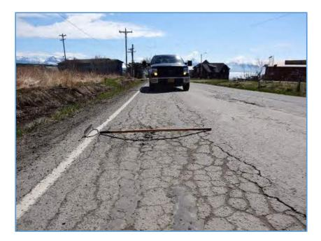
Figure 5: Extensive Alligator cracking and Rutting on Ohlsen Ln.
