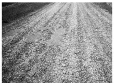
Severe raveling and loss of surface material.
