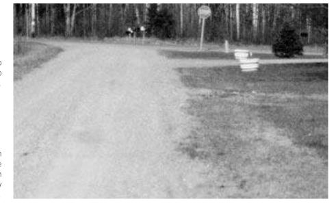
Shallow, narrow ditch cannot carry surface water causing ditch erosion and temporary roadway flooding.
