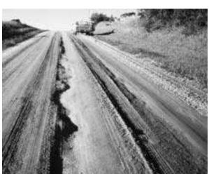
Poorly graded crown traps water causing it to run down center of road.
