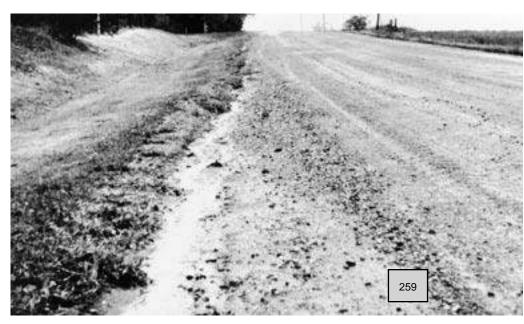
Plenty of crown and excellent ditch. Needs routine grading to eliminate slight secondary ditch and loose gravel.
