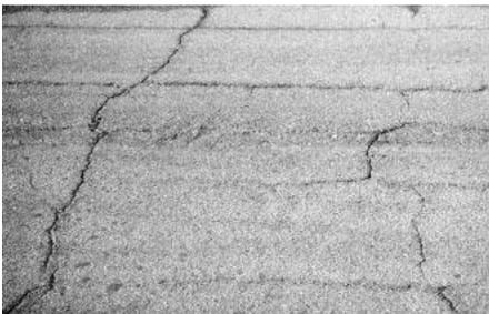
Extensive block cracking in an irregular pattern.
