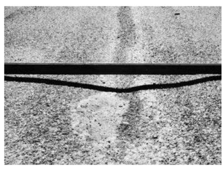
A Rut in wheel path needs regrading to eliminate ponding and prevent further road deterioration.
