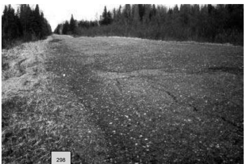
Severe frost damage. Reconstruct.
