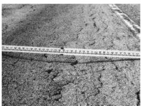
▲ Severe rutting. Strengthen base and reconstruct.
