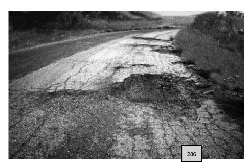
Large, isolated pothole, extends through base.
