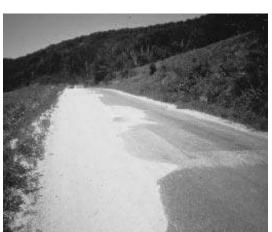
Wedges and patches extensive but in good condition.
