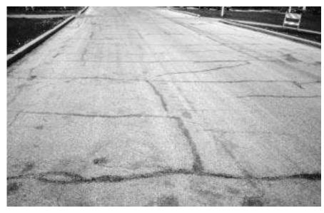
Intermediate-size block cracking, 1'-5' across with open cracks.
