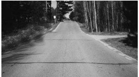
Tight and sealed transverse and longitudinal cracks.
