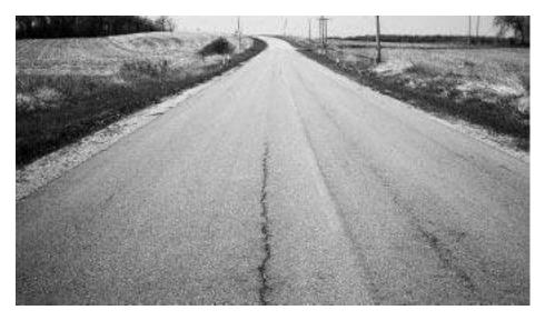
Longitudinal cracking; early load-related distress in wheel path.
