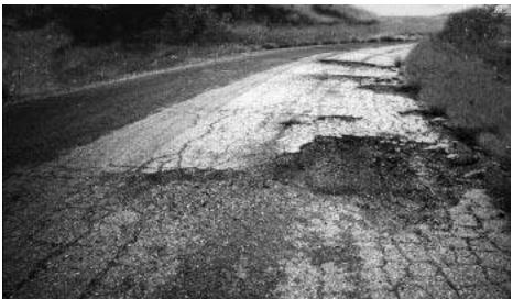
Potholes and severe alligator cracking. Failed pavement. Reconstruct.
