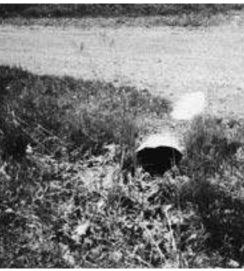
Shallow ditch and partially filled culvert. Ditch needs cleaning and culvert should be lowered to allow a minimum of 12" of aggregate cover.
