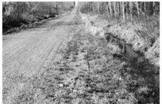
▲ Lack of ditch on right causes ruts. Needs gravel.
