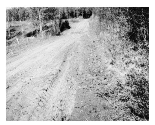
Failed — Reconstruction required Needs complete rebuilding. Travel is difficult; road may be closed at times.
