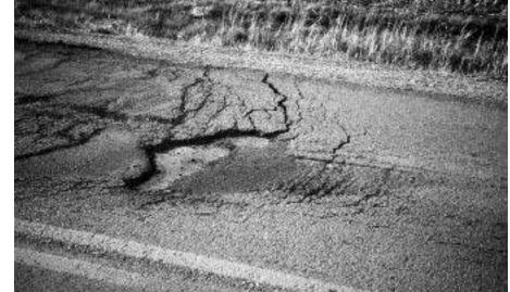
Loss of bond between pavement layers allows traffic to break loose pieces of surface.
