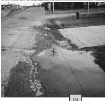
Consider both pavement surface drainage and lateral drainage (ditches or storm sewers). Pavement should be able to quickly shed water off the surface into the lateral ditches. Ditches should be large and deep enough to drain the pavement and remove the surface water efficiently into adjacent waterways.
