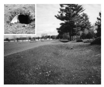
Highshoulder and no ditch lead to pavement damage. Needs major ditch improvement for a short distance. RATING: Fair
