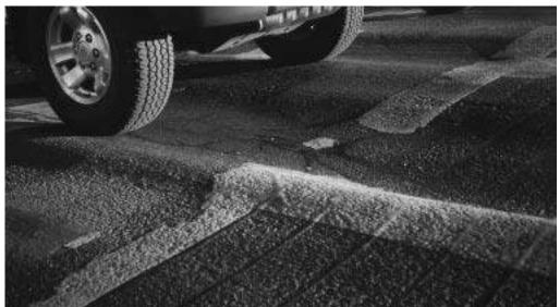
Severe rutting over 2" caused by poor mix design.
