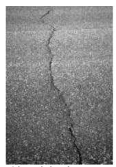
Tight cracks less than 1/4" in width.
