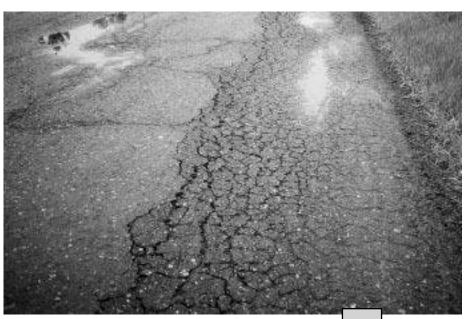
Open raveled alligator cracking with settlement along lane edge most likely due to very soft subgrade.
