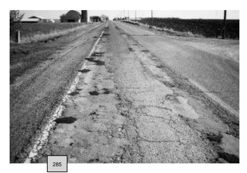
Extensive patching in very poor condition.
