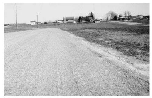
Flat crown with poor grading has created secondary ditch preventing free drainage into
