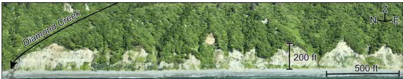
Figure 10. Looking northeast at the coastal bluffs of Diamond Creek. The bluffs are tall, exposed, and undercut, leading to higher instability. This is a screenshot from our oblique image-derived 3D model.
