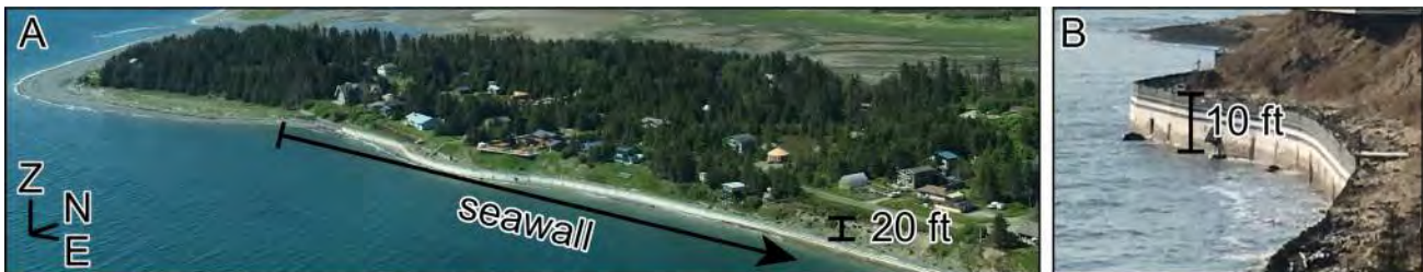
Figure 13. A. This 2019 photo looking northwest at Munson Point (left) shows the seawall protecting grassy and exposed bluffs. B. This closeup photo shows how water comes right up to the seawall and would surely undercut the bluffs.
