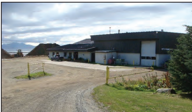
City of Homer existing Public Works facility.
