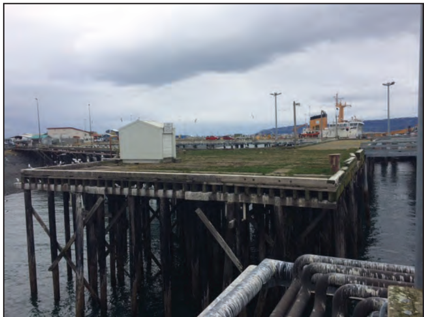
The former Main Dock in Homer's Port & Harbor is over fifty years old, defunct and deteriorated to the point that it is a hazard and a liability.
