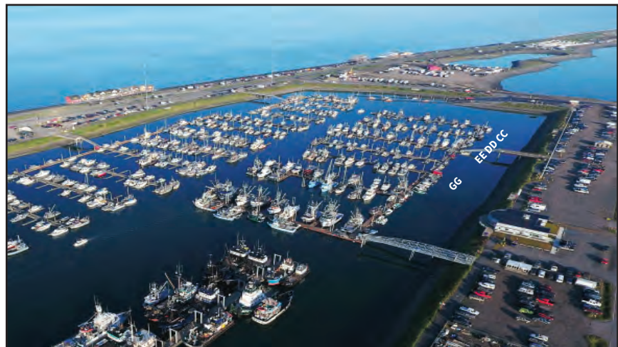
System 4 ramps to be replaced next.
