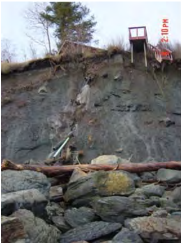
Photo 2: Homer Bluff erosion December 2006
