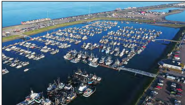
System 4 floats to be replaced.
