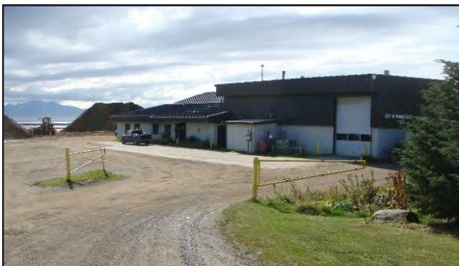
City of Homer existing Public Works facility.
