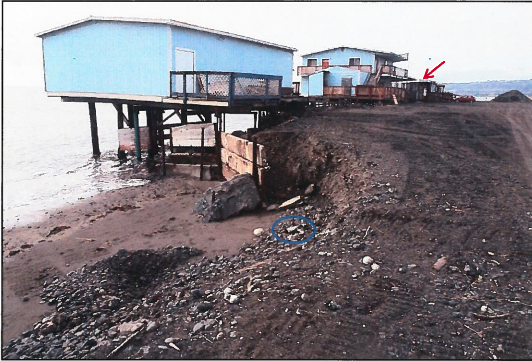
Annually the height of the parking area in front of the buildings has to be filled in. The Glacier Drive In, adjacent NW, is partially visible at arrow.
