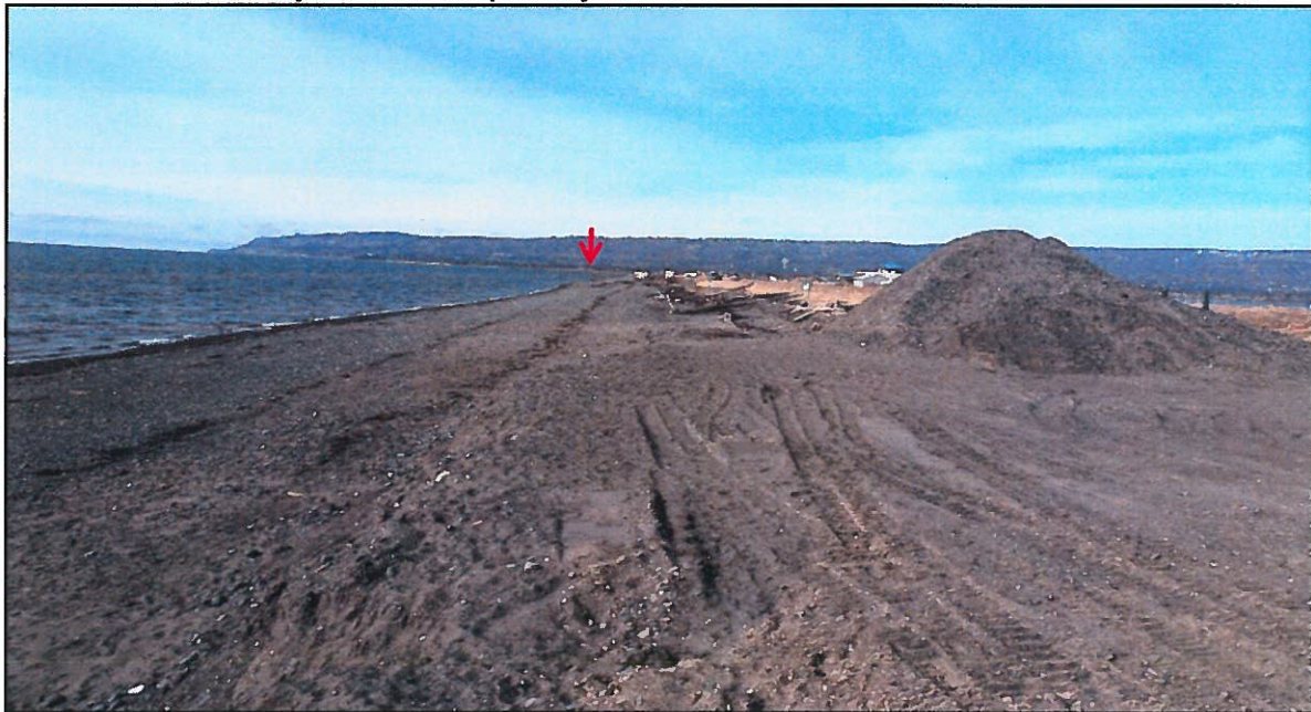
Looking toward the Homer mainland from the edge of the Glacier Drive In parking area. The pole at arrow was formerly above tide level, part of the RV site improvements on Lot 3, Homer Spit Three S/D. This area of the Spit has been severely impacted by erosion.
