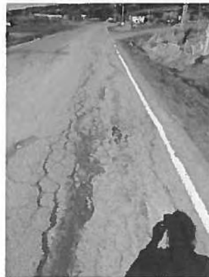
Cracking and pothole formation on Ohlsen Ln. Narrow road corridor causes out of spec travel lanes, shoulders and
