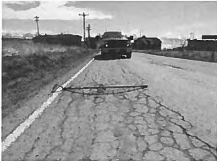
Ohlsen Ln: Paved road with multiple issues including major cracking, subsidence, and out of spec road corridor
