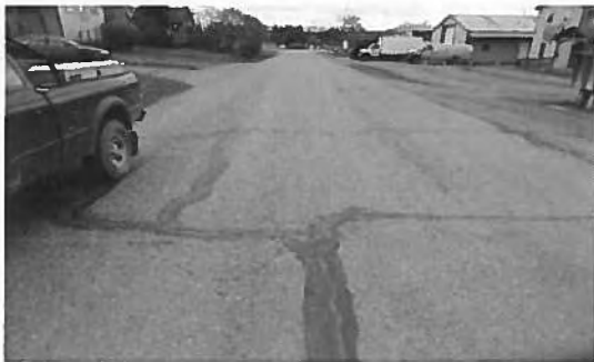
Extensive crack repair on Grubstake Ave. (West) Crack sealing is an annual maintenance task
