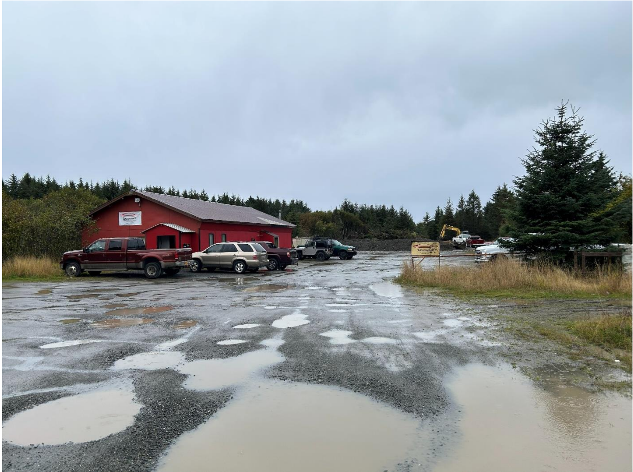
Existing building slated for demolition located at 3145 Lampert Lane
