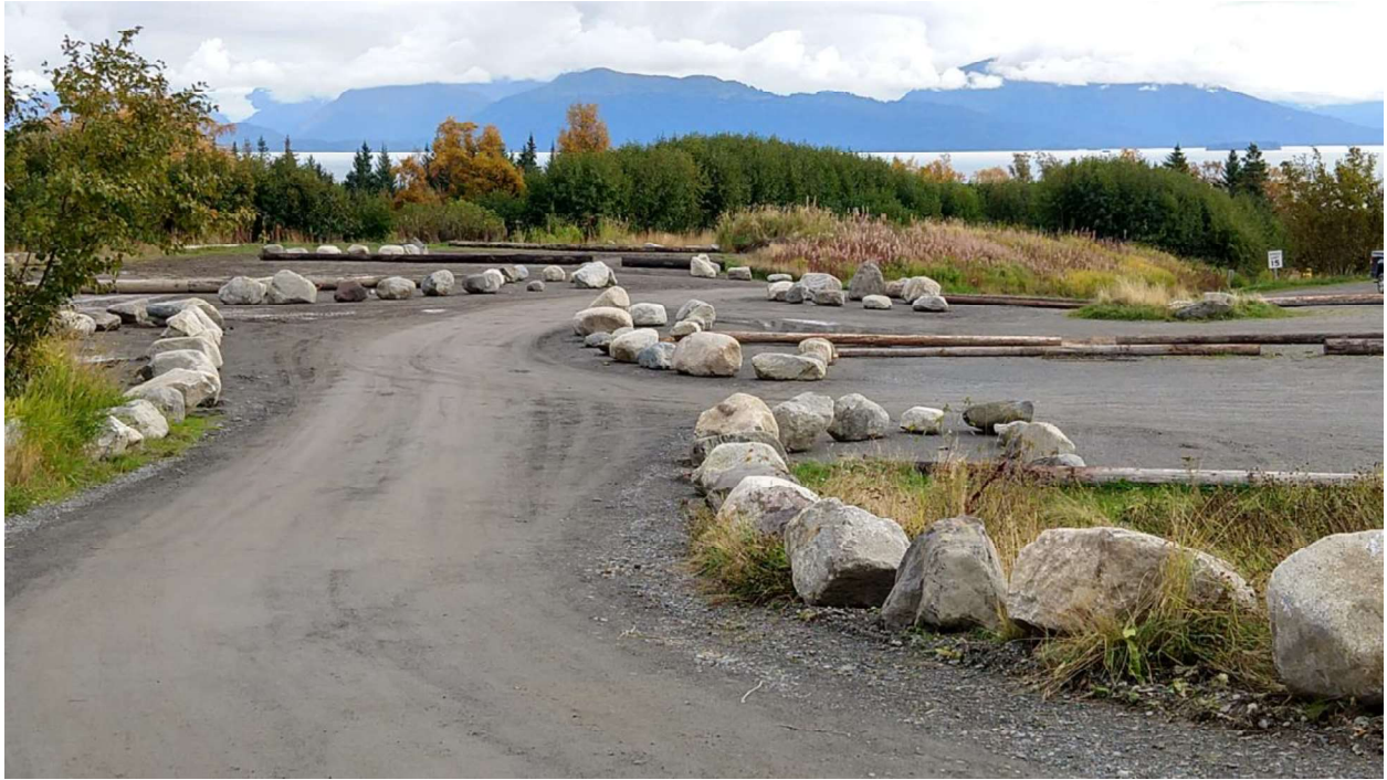
Looking south down the new access road realignment
