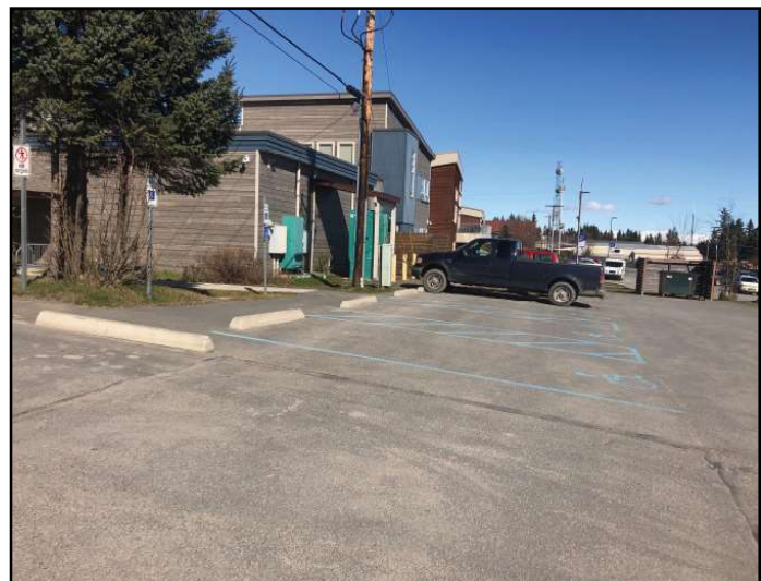
The cross slope of the accessible parking spaces at the lower entrance to City Hall exceeds the maximum allowed.
