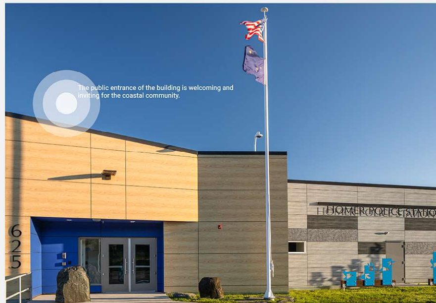
Blue backdrops at entrances bring the deep blue ocean from Kachemak Bay into the building
