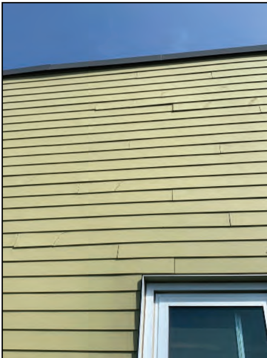
Examples of damaged and broken siding on the library's south-facing wall (at left) and above the library's back door (at top).
