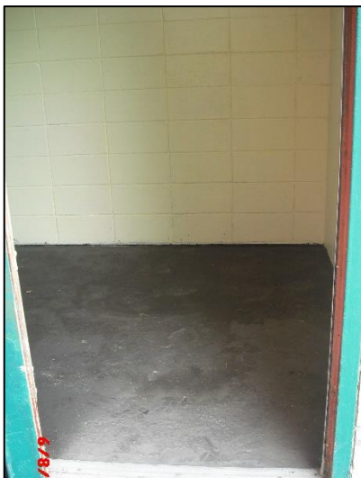
2019 floor paint reapplication already damaged due to leaking roof
