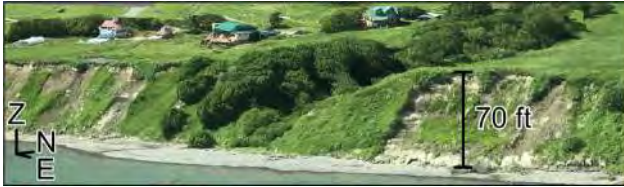
Figure 15. Looking west toward the grassy-to-exposed bluffs and a densely vegetated creek near East End Road in the oblique image-derived 3D model. Exposed slopes show groundwater flow.
