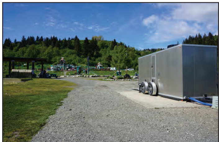
A permanent public restroom facility is needed to replace the temporary mobile restroom facility at the park.
