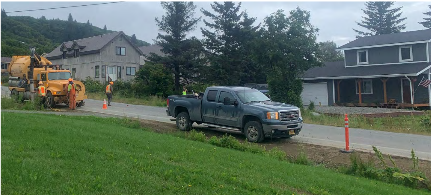
Crews working on the Main Street Sidewalk on July 19 th
