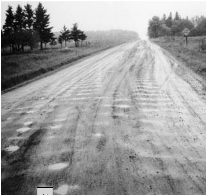
► Severe washboarding traps water.
