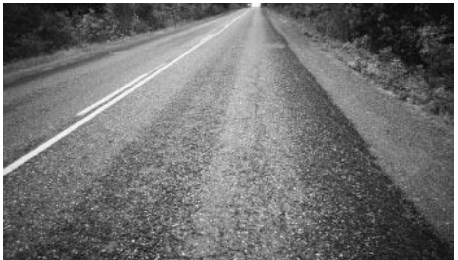
► Moderate to severe raveling in wheel paths.
