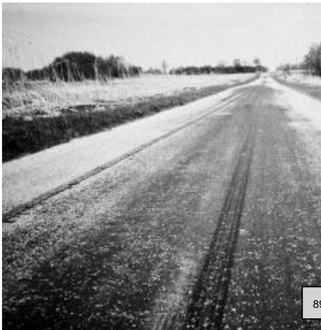
▼ Severe flushing.
