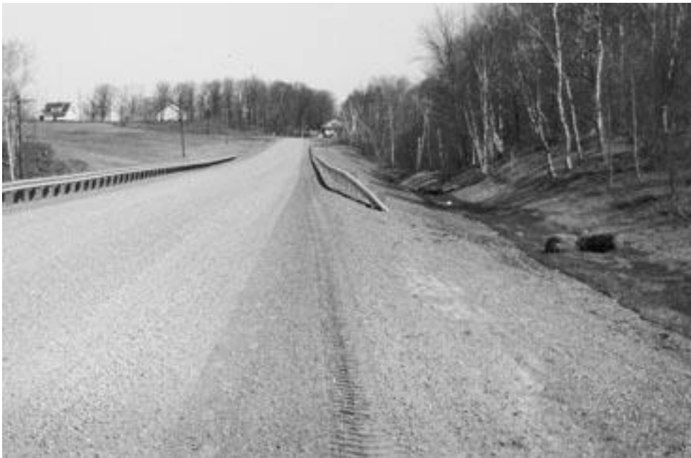
Partial drainage. Ditch and new culvert being added on left. Little or no drainage on right.
