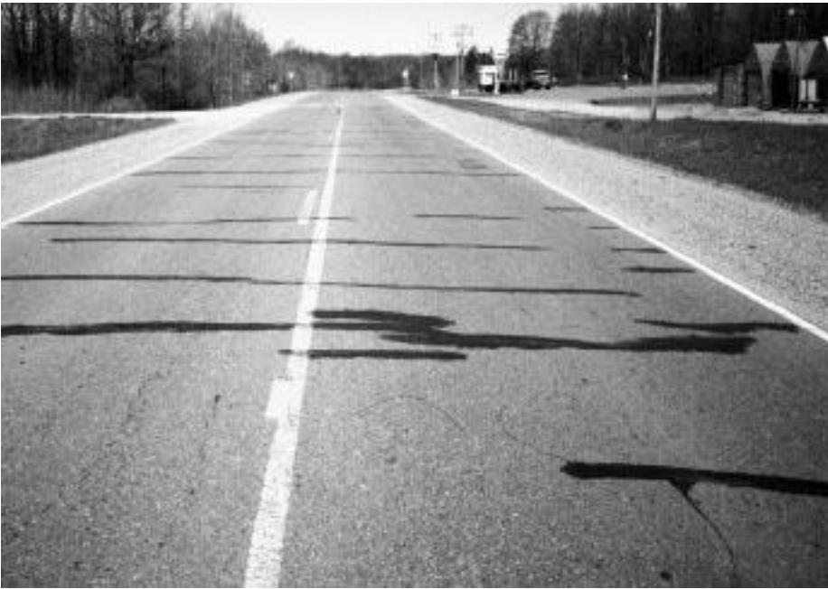
◀ Sealed cracks, a few feet apart.
