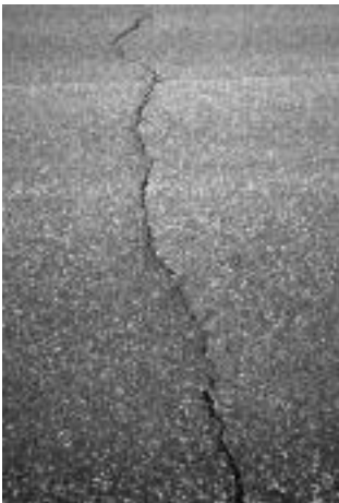
▲ Tight cracks less than 1/4" in width.
