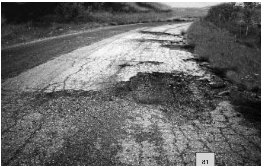
◀ Large, isolated pothole, extends through base.
