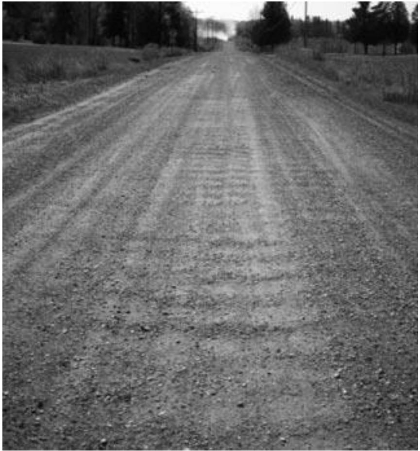
▼ Moderate washboarding in center of road.
