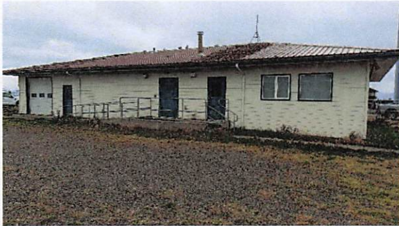
USCG Cutter Support Building
