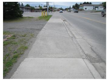
Figure 20 : Driveway Entrance with Steep Cross Slope
