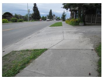
Figure 19: Driveway Entrance with Level Cross Slope
