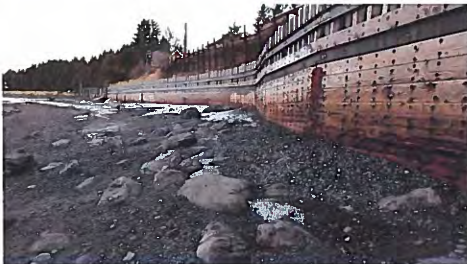
Figure 3 - January 2019 West Portion of Wall
