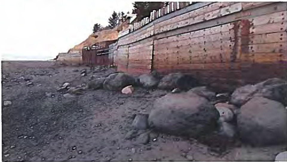
Figure 2 - January 2019 East Portion of Wall
