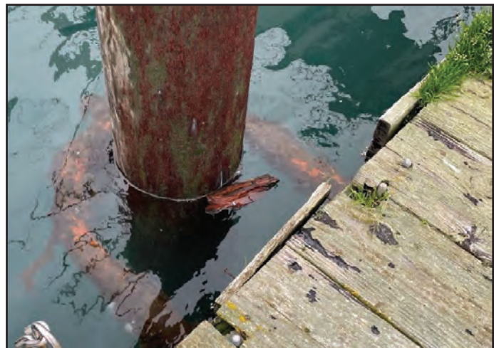
Low freeboard resulting in submerged pile collar.
