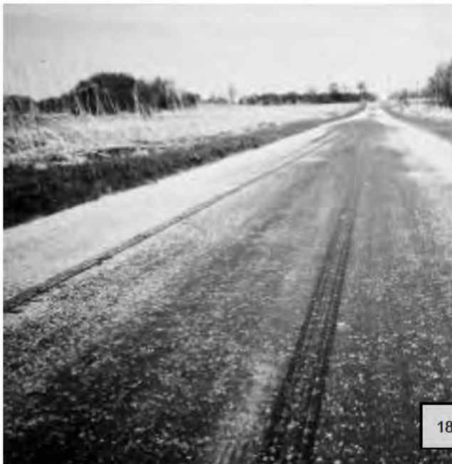
▼ Severe flushing.
