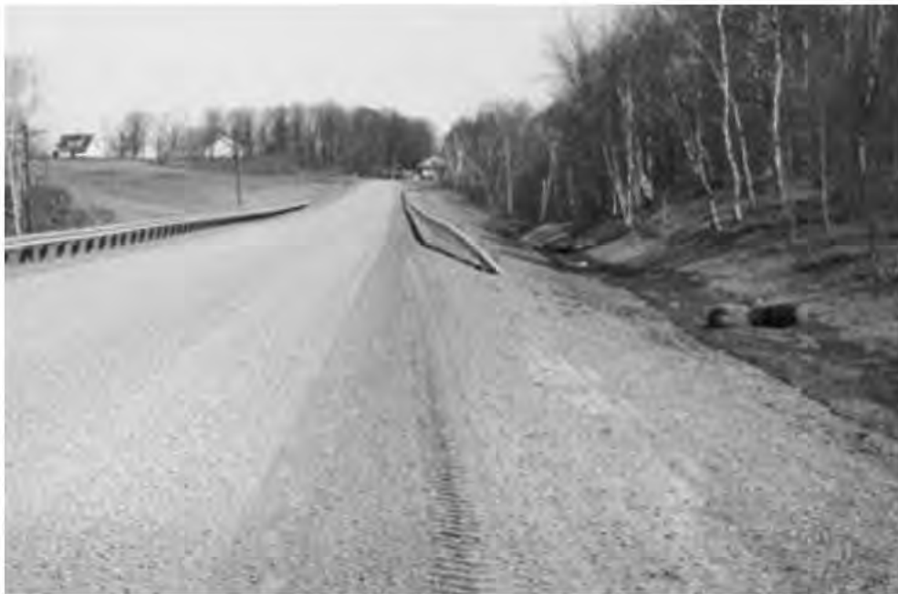
◀ Excellent drainage with wide deep ditches.
