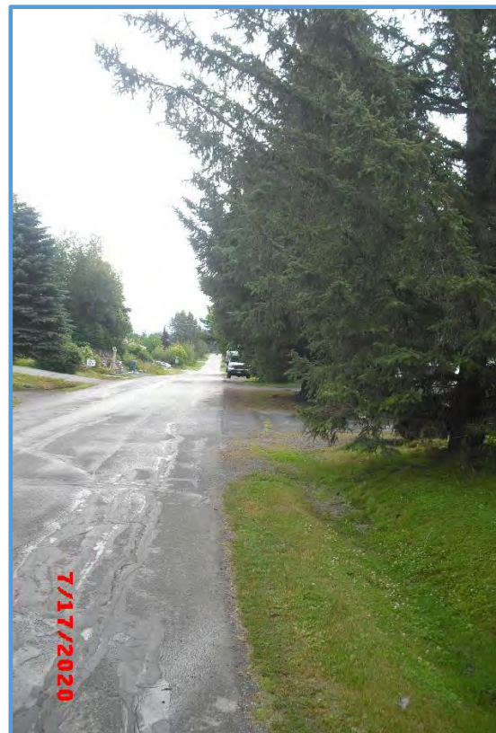
Figure 8: Tree limbs within roadway
