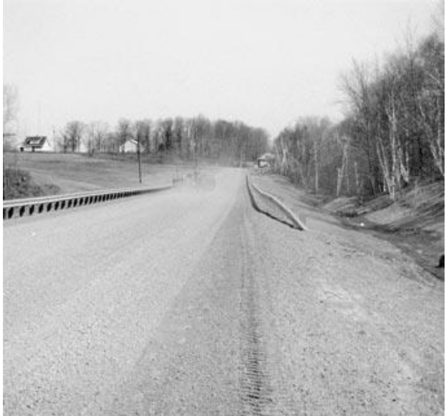
► Newly constructed road with excellent crown, drainage and gravel layer.
