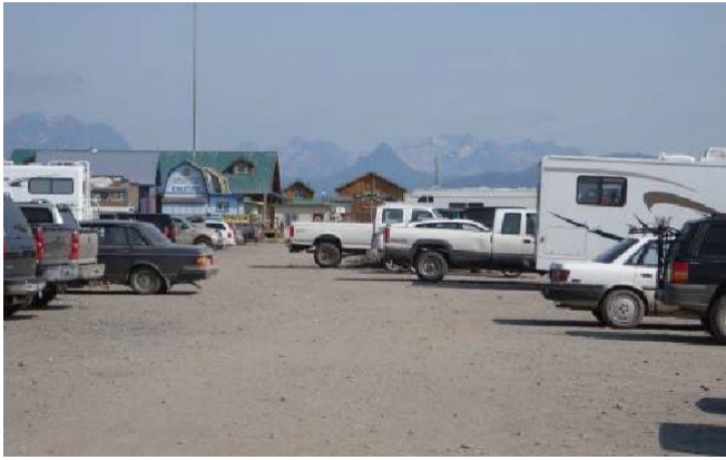
Unmarked gravel lots create some unique parking patterns. As currently configured they also tend to drain poorly and become riddled with puddles when it is rainy.
