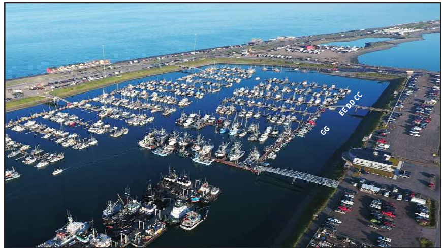
System 4 ramps to be replaced next.
