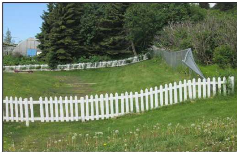
Though charming, the white picket fence that surrounds Bayview Park is in need of constant repair. A more practical chain length fence is needed to keep young children out of roads and ditches.
