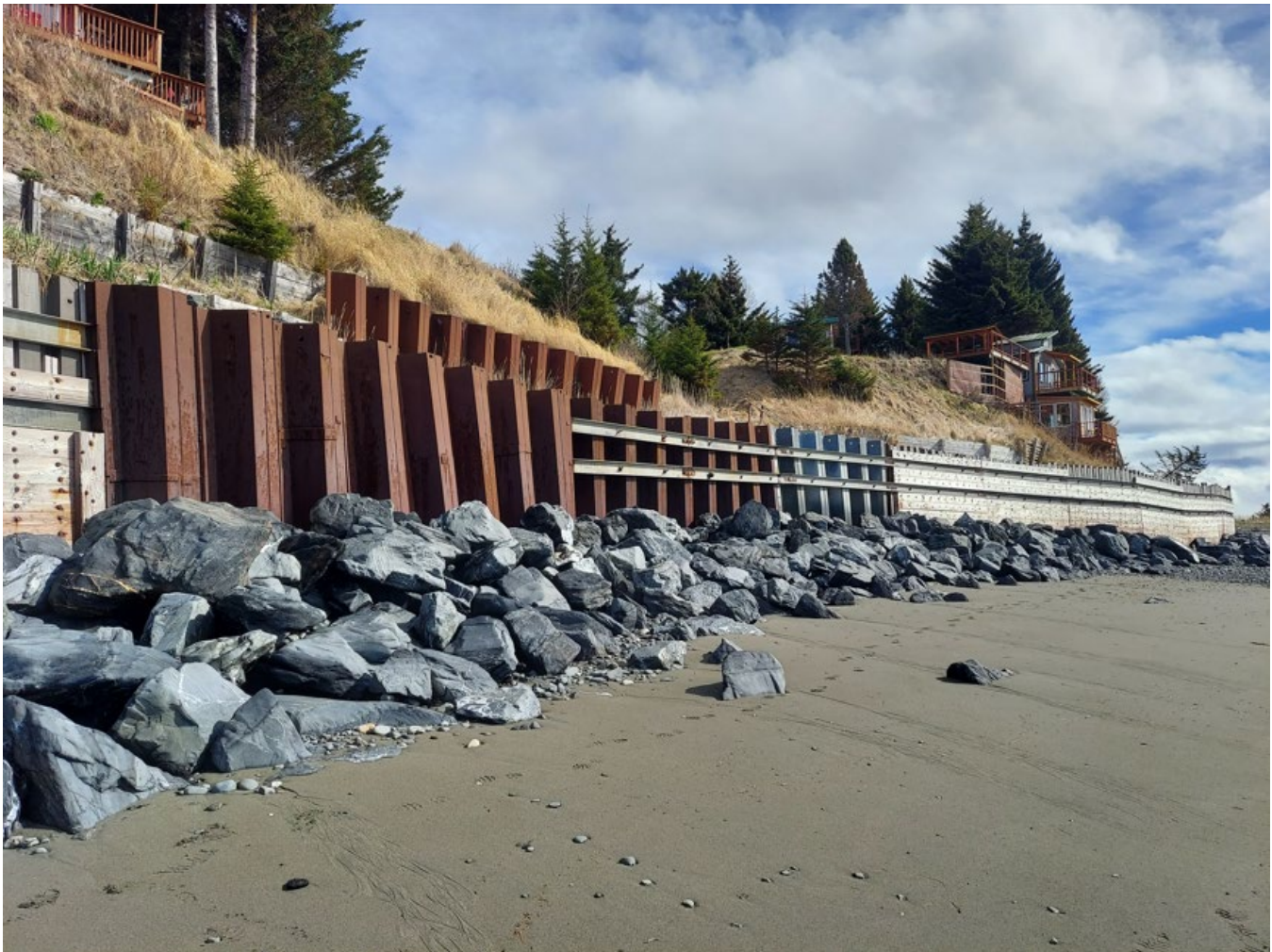
This photo shows a larger sheet pile repair that was done to strengthen up a sheet pile wall failure.
