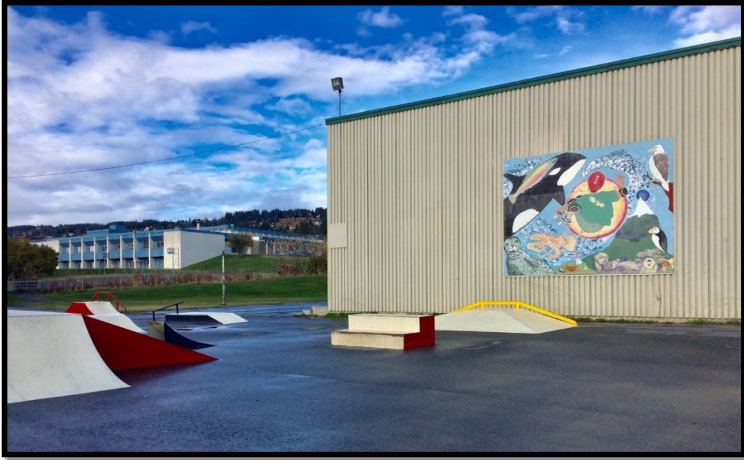
Skate Park that was constructed while the Boys and Girls Club occupied HERC-1.
