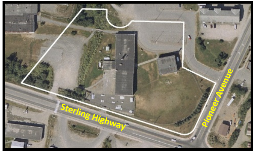
2003 photograph of the HERC property. HERC-1 (on left) is the focus of this report. HERC-2 (on right), is only discussed in terms of demolition costs.
