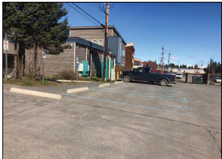
The cross slope of the accessible parking spaces at the lower entrance to City Hall exceeds the maximum allowed 1:48 under ADA standards.
