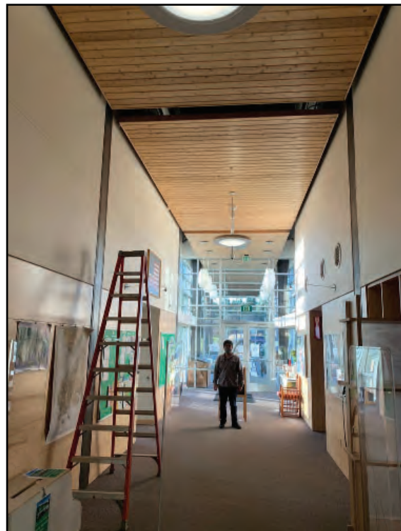
Structural frame for a security gate that was built in to the Library's entry hall.
