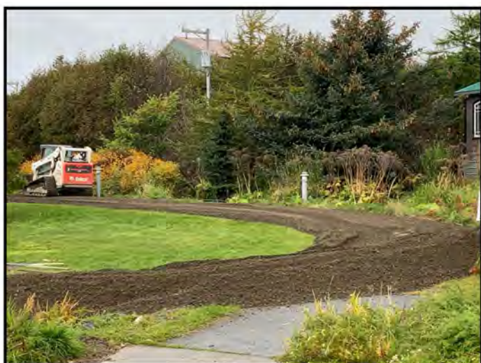
Contractors improved the surface of the Story Trail at Homer Public Library with new fabric and surface material.
