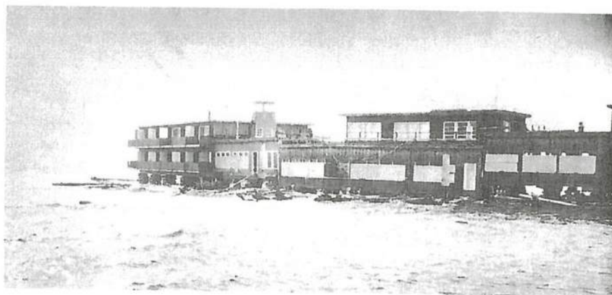
8.—Land's End Hotel jacked up 8 feet to avoid inundation by high tides. View from Homer dock looking west. View during first 20-foot tide. Middle part of hotel not yet raised.
