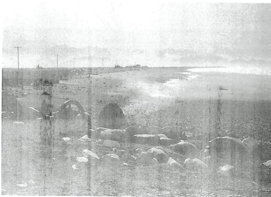
21.—Erosion on the lee side of the last of a series of four groins, a few days after the earthquake.
