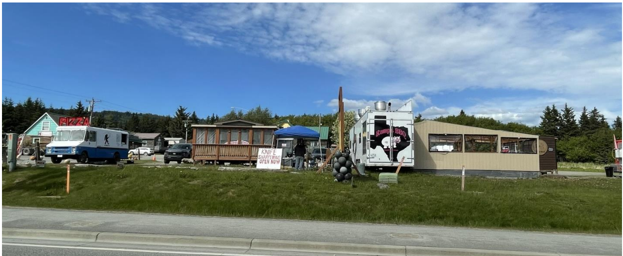
View of 3582 Main St. from Sterling Hwy. looking north.
