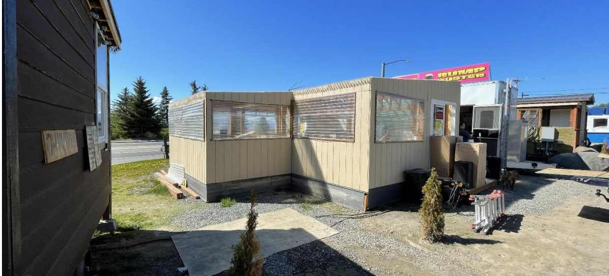
Unpermitted enclosed dining structure located 3582 Main St.
