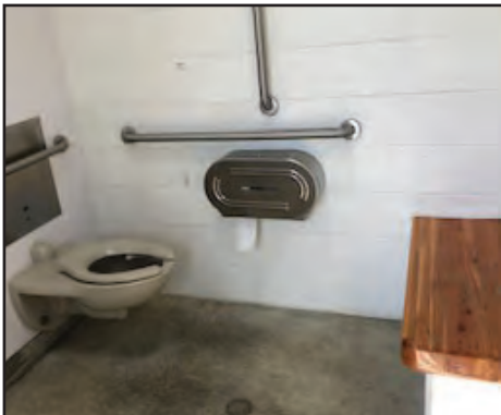
This project will correct accessibility issues at City of Homer public restrooms. Some depicted here include improperly placed dispensers and grab bars, lack of wheel chair space from bench, incorrect door swing and lack of cover on the lower pipes
