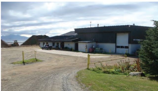
City of Homer existing Public Works facility.
