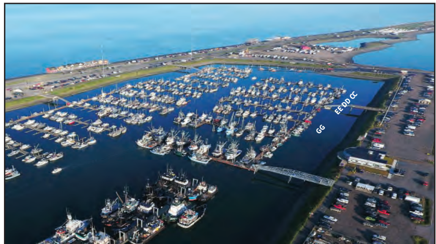
System 4 ramps to be replaced next.
