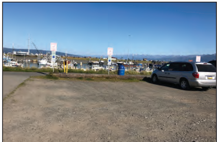
Accessible parking spaces at Ramp 4 in the Port & Harbor provide an example of where spaces need to be paved and a path of travel provided to the sidewalk.
