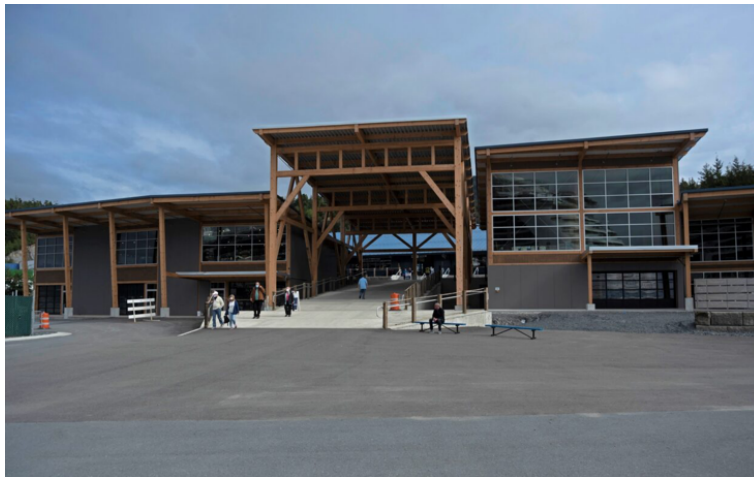
Juneau-based architects Jensen, Yorba, Wall designed the 40,000 square foot Sitka Sound Cruise Terminal. The timbers were pre-fabricated offsite, and assembled in Sitka. Inside the facility a retail store is already open. Soon to come: A taproom featuring local beers, and a seafood restaurant. (KCAW photo/Tash Kimmell)
