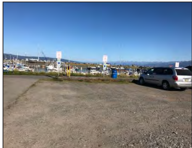
Accessible parking spaces at Ramp 4 in the Port & Harbor provide an example of where spaces need to be paved and a path of travel provided.
