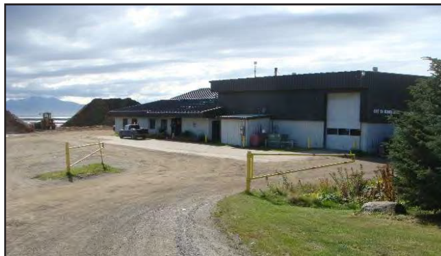
City of Homer existing Public Works facility.
