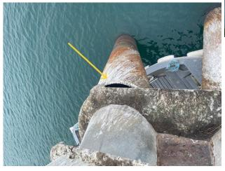
(Complete separation from piling cap and failed weld)
