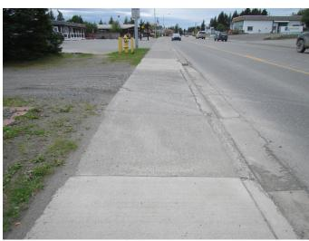
Figure 20 : Driveway Entrance with Steep Cross Slope
