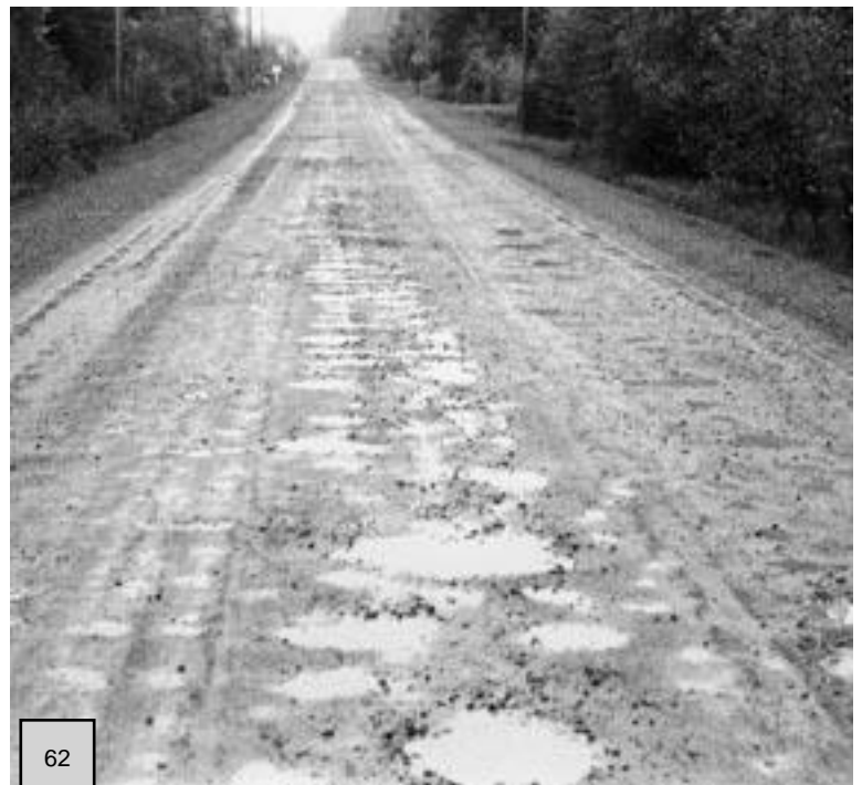
No crown, poor drainage, and ▼ needs gravel.
