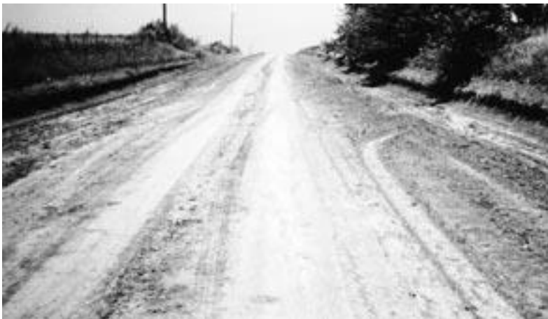
▲ Little gravel and almost no ditches or crown.
