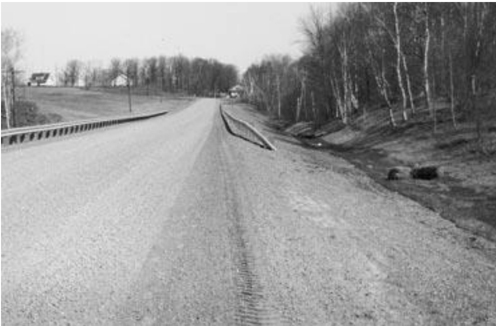
◀ Excellent drainage with wide deep ditches.
