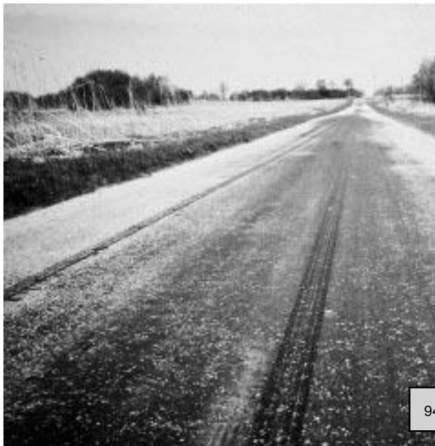
▼ Severe flushing.
