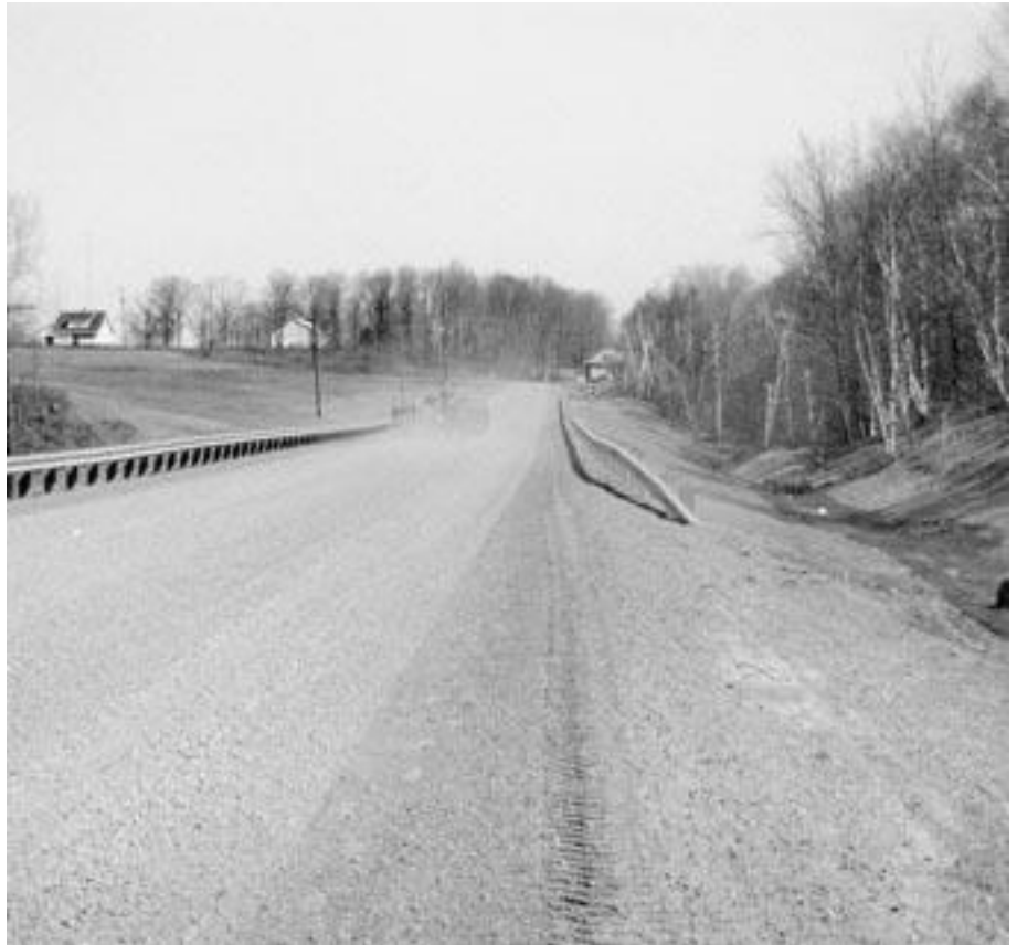
► Newly constructed road with excellent crown, drainage and gravel layer.
