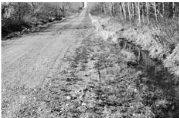
No crown, poor drainage, and ▼ needs gravel.
