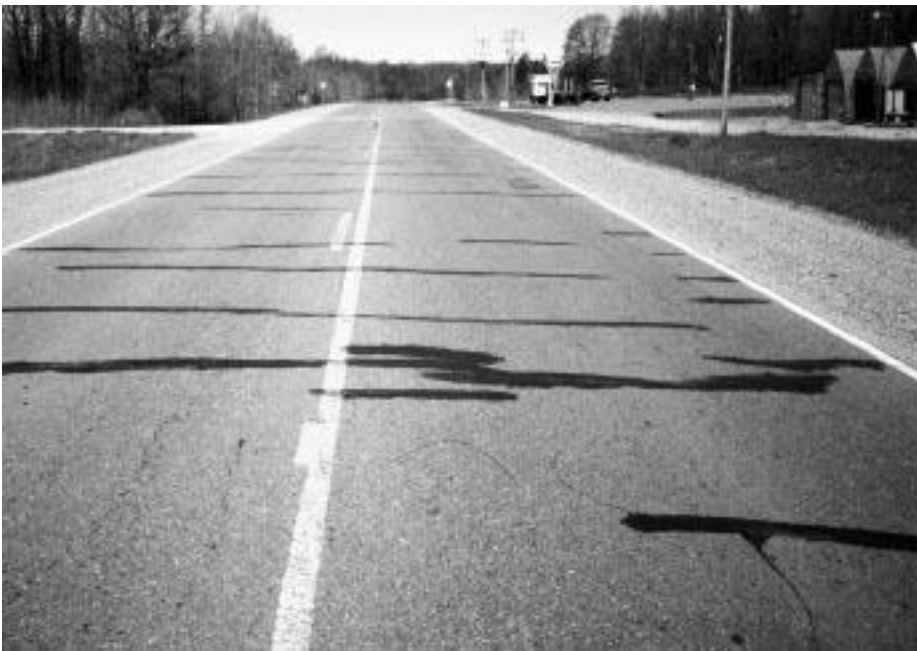
◀ Sealed cracks, a few feet apart.
