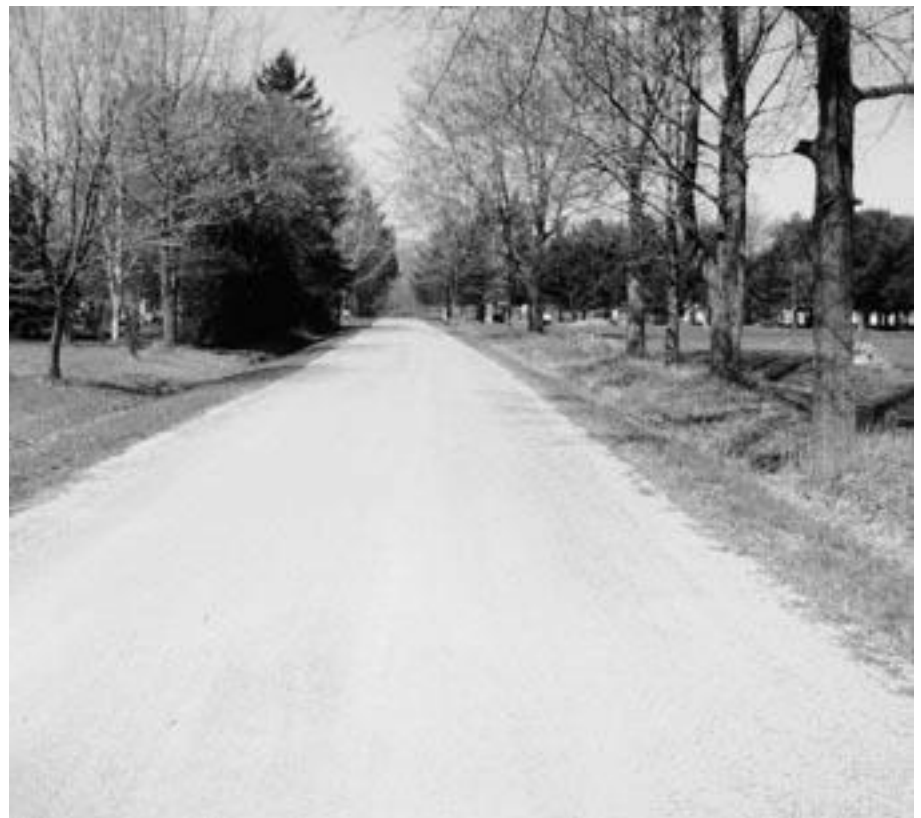
► Road has excellent crown. Gravel has been stabilized for dust control. Very good drainage.
