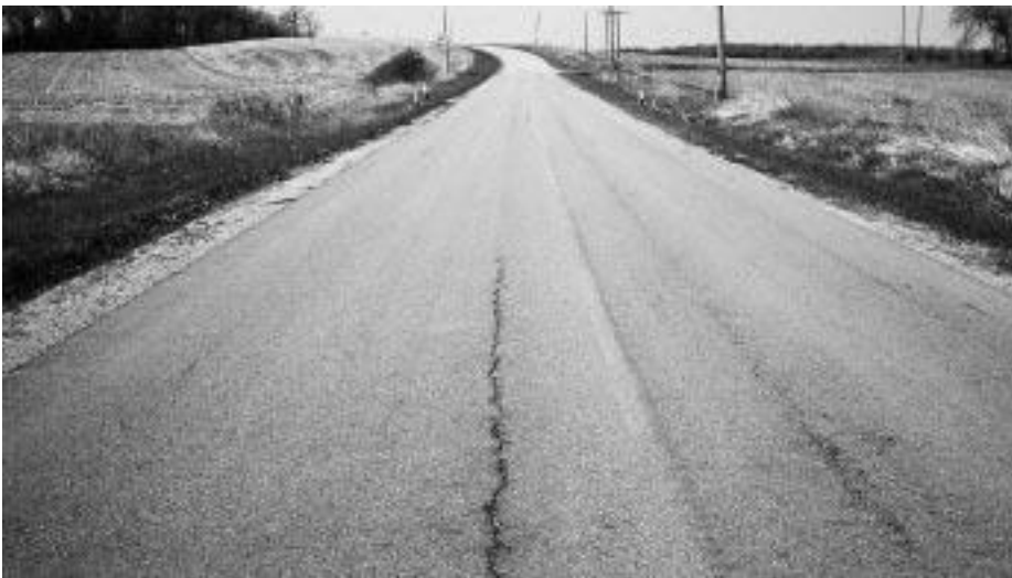
▼ Slight rutting; patch in good condition.
