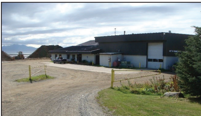
City of Homer existing Public Works facility.
