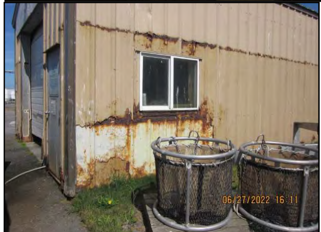
Corrosion is compromising the Fish Grinding building's structural integrity and degrading interior fixtures.
