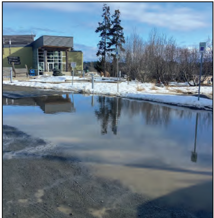
Poor drainage across Homer Public Library's sloped parking lot, especially during winter and spring freeze thaw cycles, creates hazardous walking conditions.
