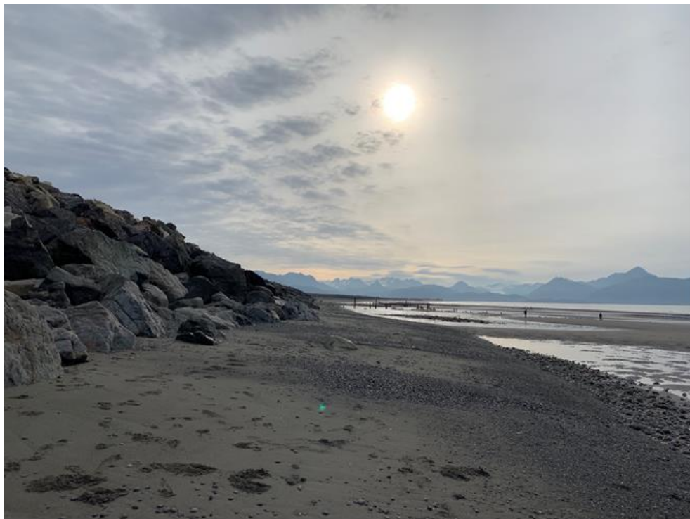
Figure 3. Condition of USACE revetment along the Spit.
