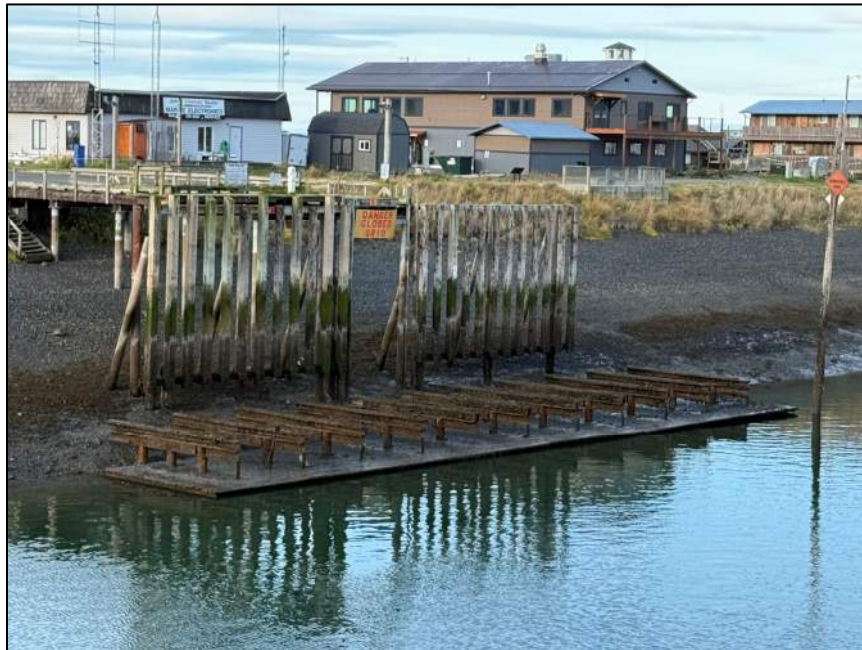
Figure E.1. Homer Harbor Steel Grid (low tide)
