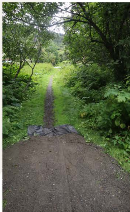
Calhoun resurfacing in progress shows the difference between the old trail and the new one. Photo credit: Matt Steffy
