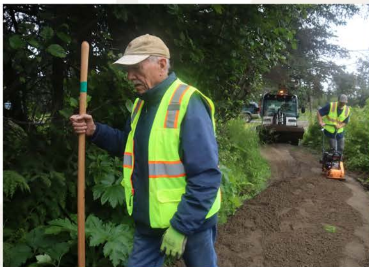
Volunteer Mike Haines smooths out new gravel that City Parks staff Chad Felice delivers with the Toolcat while Matt Hornaday runs the compactor on Calhoun Trail. Photo credit: Matt Steffy
