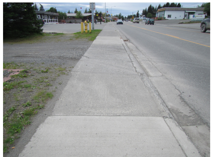
Figure 20: Driveway Entrance with Steep Cross Slope
