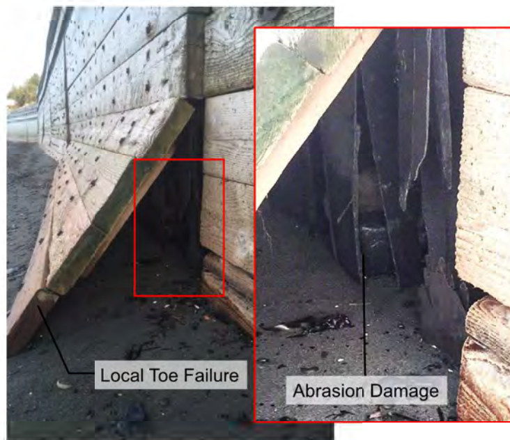
Figure 4. Example of observed local failure – correlates to sink hole at top of the seawall. Inset shows previous assumed abrasion damage.
