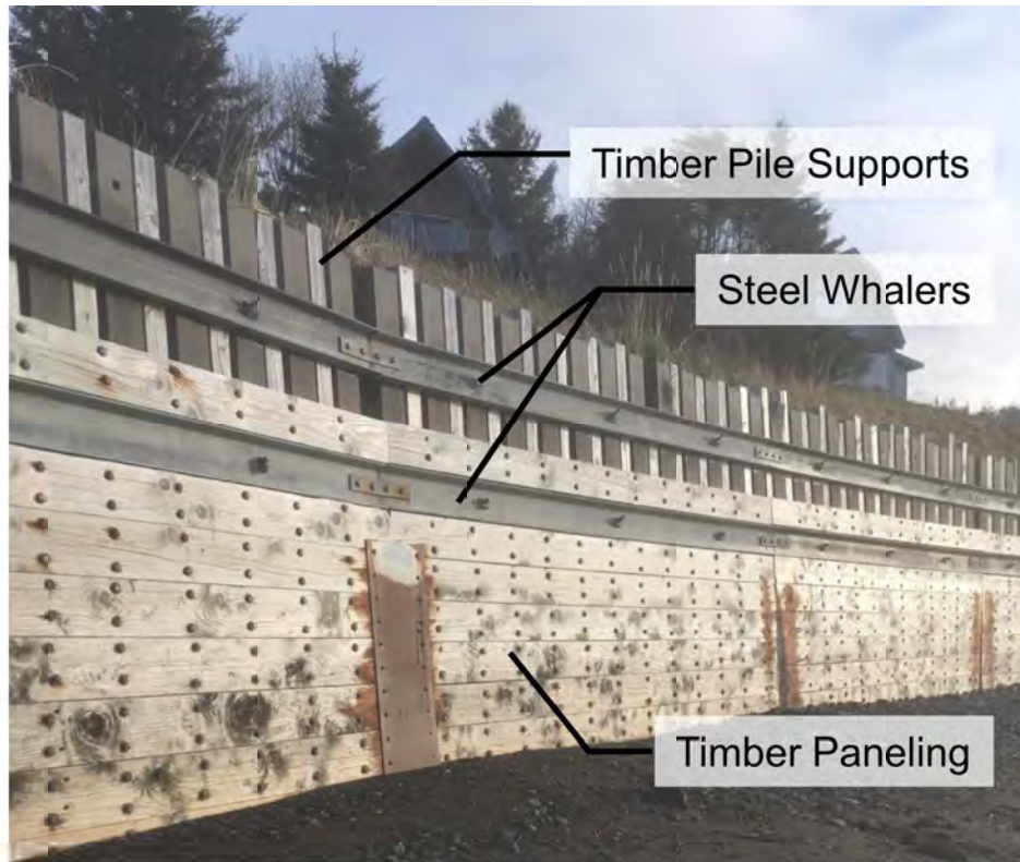
Figure 3. Seawall existing condition.
