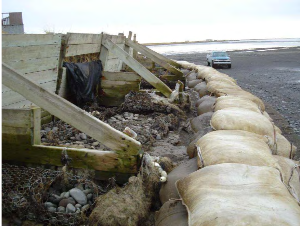
Figure 10. Example of geotextile container revetment (pyramid layout). In the Homer seawall case, the containers would be placed against the seawall.
