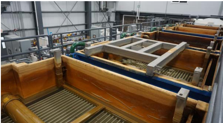
Membrane Filters at Water Treatment Facility
