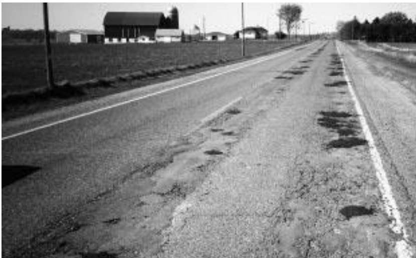
▲ Patches in poor condition, wheelpath rutting. Pulverize, strengthen and reconstruct.
