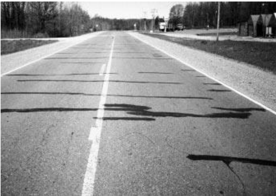
◀ Sealed cracks, a few feet apart.
