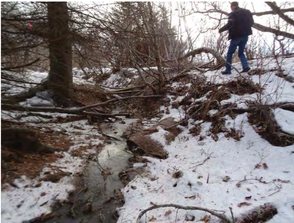
This photo looks west along Nelson Avenue and shows that surface water ran down the center of Nelson Avenue prior to culvert removal.
