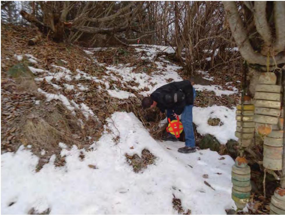
This photo looks north at the downstream end of the culvert that was removed.
