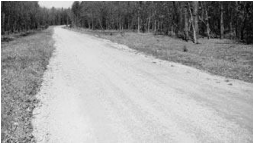
◀ Adequate gravel layer. No ruts or potholes.
