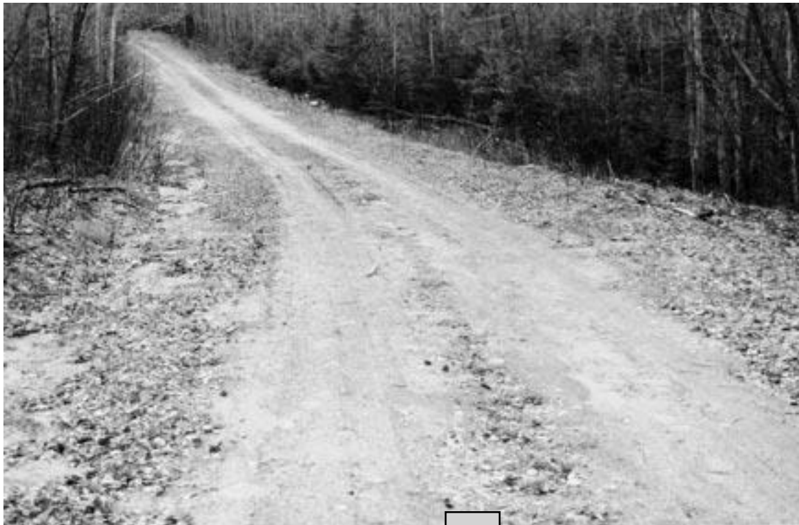
◀ Adequate gravel layer. No ruts or potholes.
