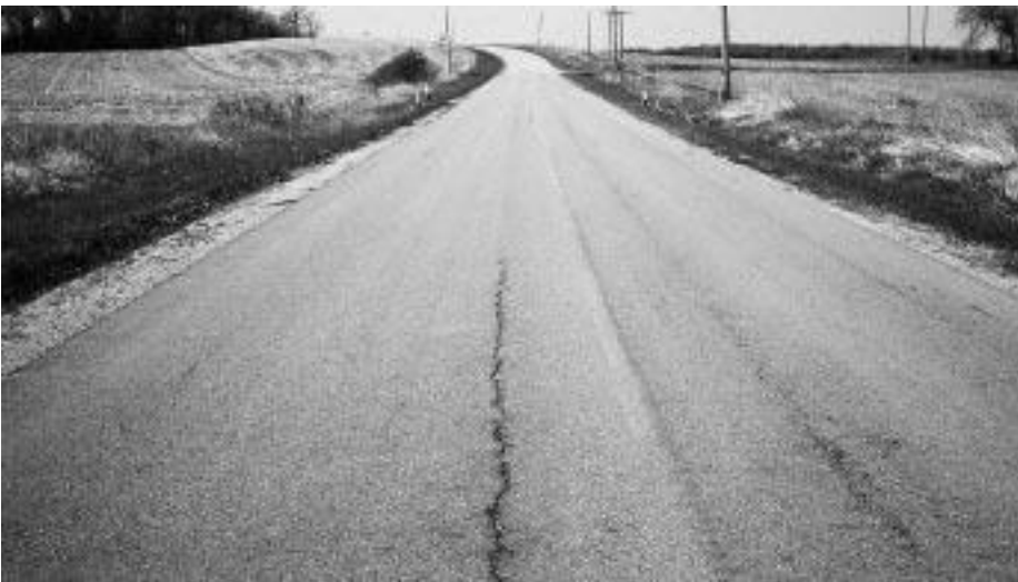
▼ Slight rutting; patch in good condition.
