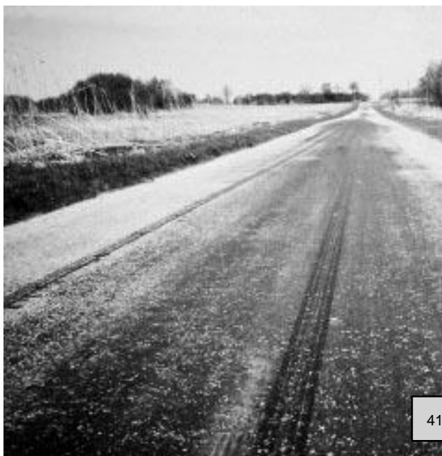
▼ Severe flushing.
