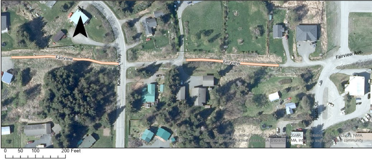
East Fairview & West Fairview-redone with new fabric and material by contractor
