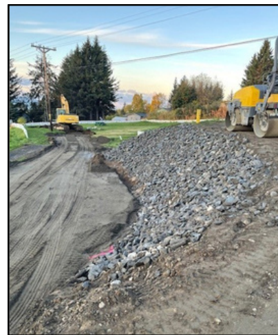
Riprap installation along the new pathway to combat erosion.
