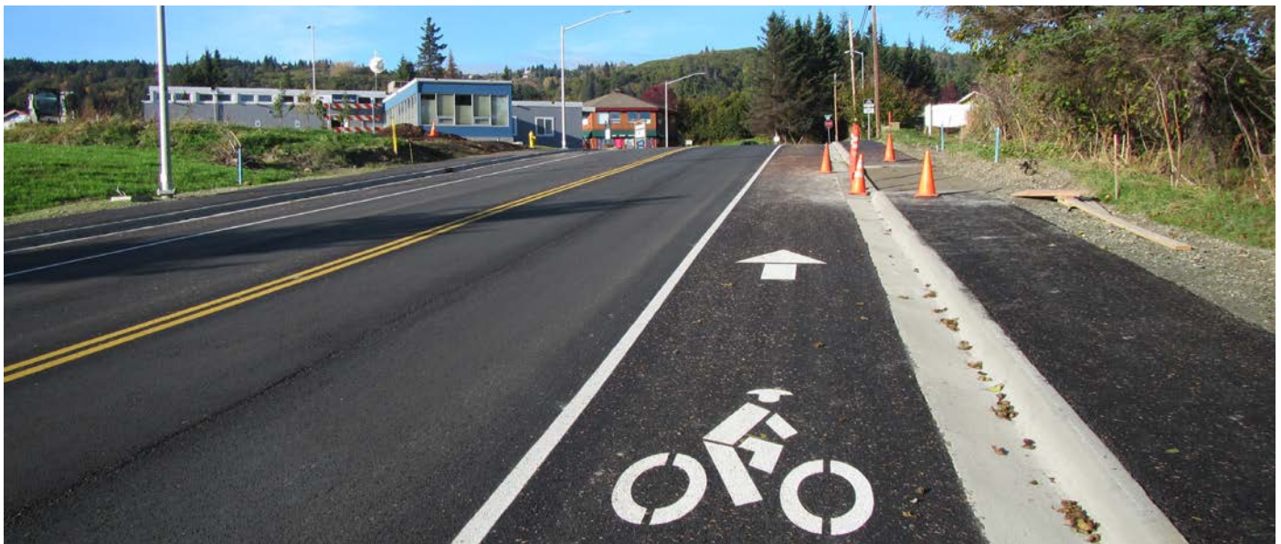
Figure 16: Greatland Street Improvements were a HART funded project in 2017.
