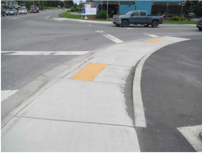
Figure 18: Curb Ramps that Direct the User into the Crosswalk
