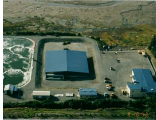
Sewer Treatment Plant (1990)
