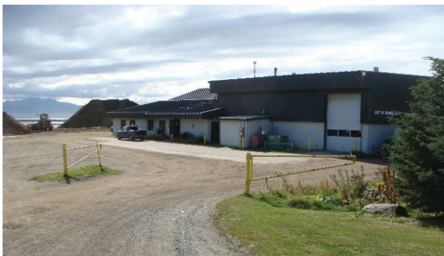
City of Homer existing Public Works facility.
