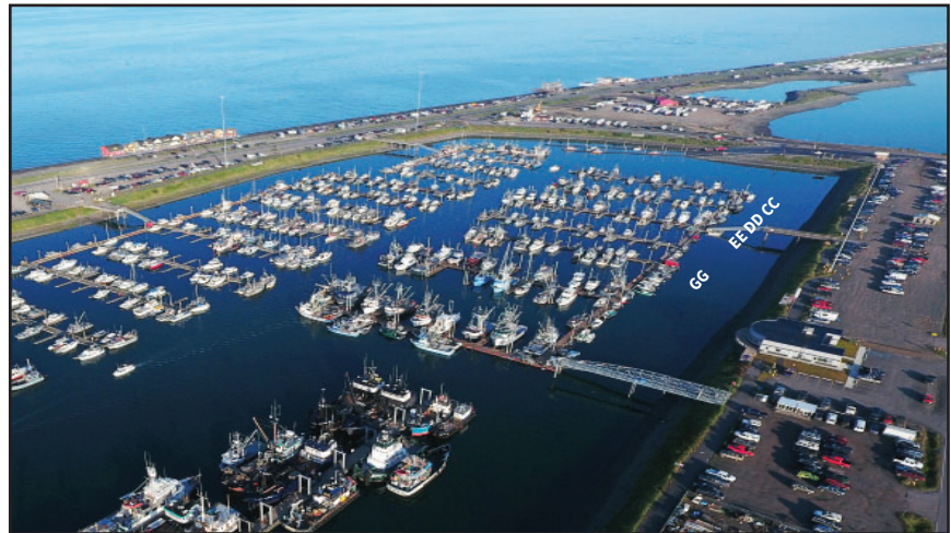
System 4 ramps to be replaced next.
